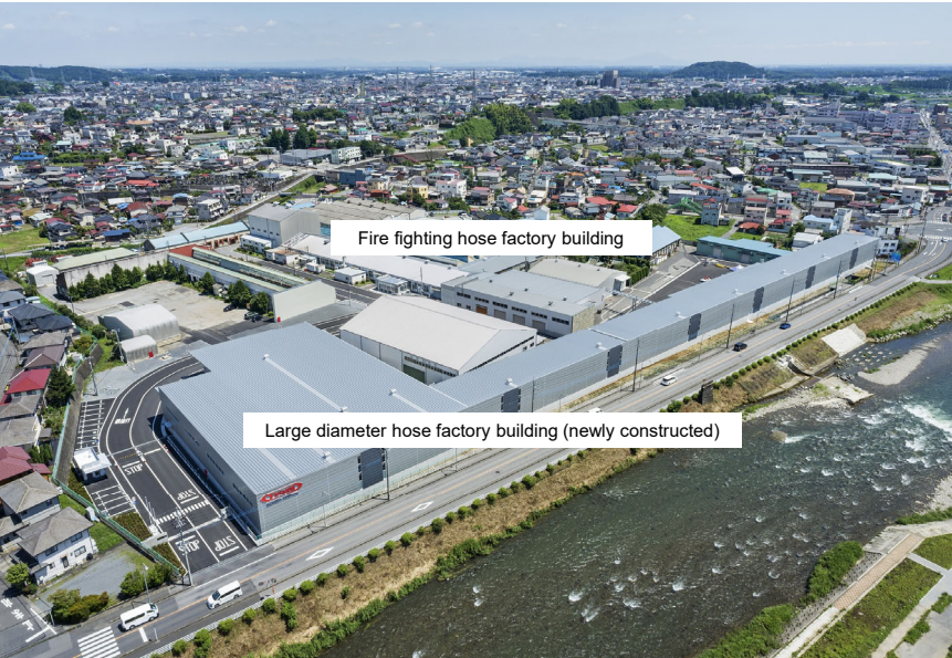
Solar panels to be installed on the new factory building (scheduled to begin operating in April 2023)
