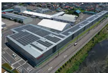
• Solar power generation system at the Kanuma Plant (since 2023)
